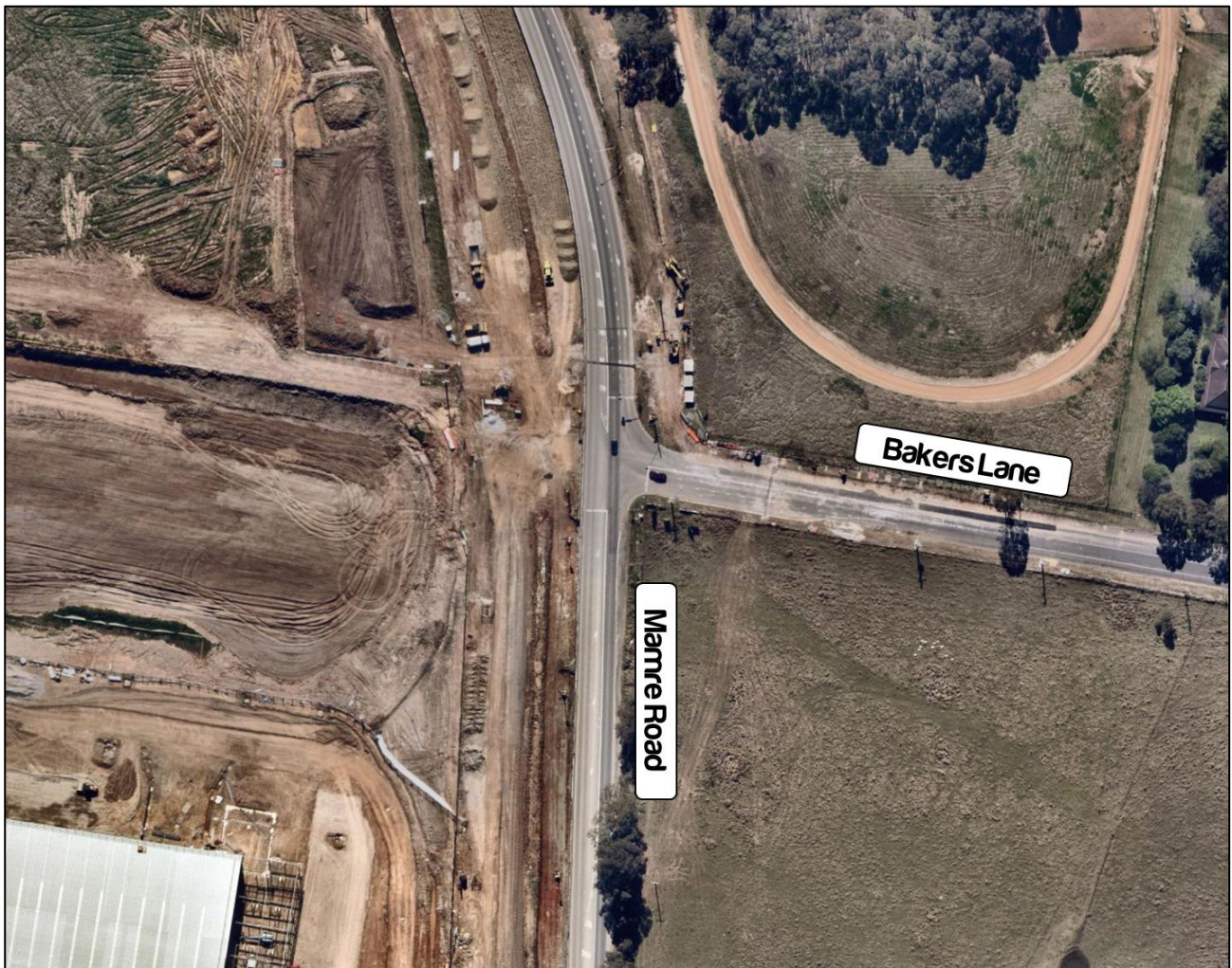
Figure 9: Existing Intersection of Mamre Road / Bakers Lane
